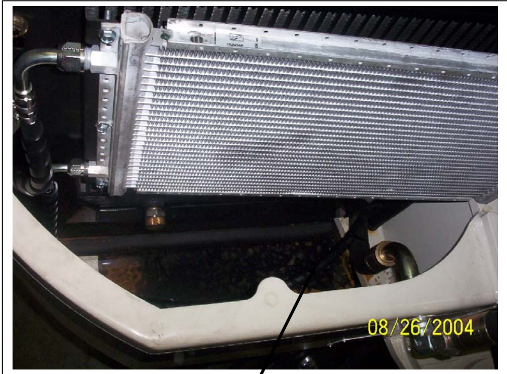
5/16" line from the lower fitting on the condenser running into the engine compartment area beside a hydraulic hose.
